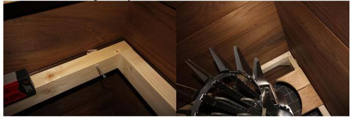
4. Place the backrests in position. The installation height is usually 400 mm - 450 mm, depending on the model and the material. This height can be raised or lowered according to your own preference. Also consider the windows! Use the window to check the installation height, if the window is positioned low in the sauna! Check the straightness with a spirit level. (Screws 55 mm long, included in the delivery!)
