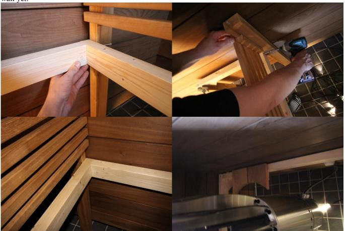
3. Lift the upper bench frames to their places. The upper bench is fitted to the metal pins on the feet by its lower edges.
