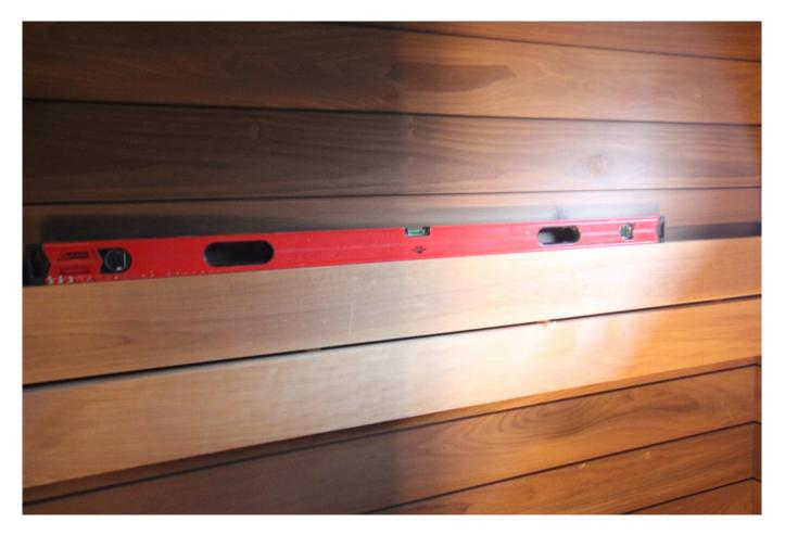
5. Place the spacers of the lower bench in position. If the spacer is on top of the joist hanger, it does not have to be fastened with screws. The joist hanger solution makes sauna cleaning easier, when you can simply lift the frames out of the way during cleaning. PLEASE NOTE! If the solid frames by the walls are long (more than 600 mm), screw them also to the walls, in the same way as the upper benches. Check the straightness with a
