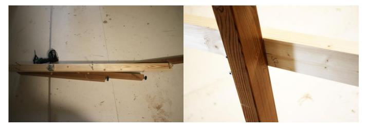
2. Connect the solid frame parts of the lower bench to the lower bench frames. (On the sample frame image, R1, R3, R4 etc.) The screws will be tightened behind the lower bench frame. Do not screw the structure to the wall yet.
