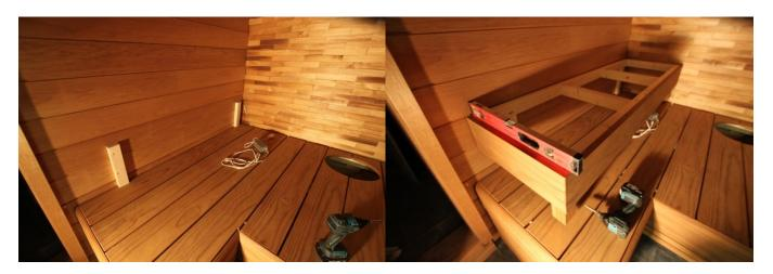
6. If your bench is opposite-facing as shown on the image, it is recommended to make sure that the sides are at the same height. Lift the top elements of the upper bench in position. Then, put the backrest in its place. The height of the upper edge is usually 400 mm from the top of the upper bench. This can be changed according to your preference.
