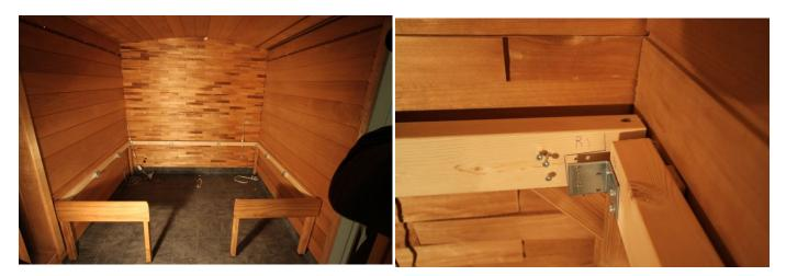
2. Place the bench skirts underneath the end board **IF** there is a glass wall in the sauna, and you want it to have a skirt. The foot/end board will have markings for its correct position.
