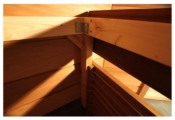
3. Place the spacers between the frames. When the spacers have been positioned correctly, centre the bench in the sauna, adjust the frames using the levelling feet, and screw the outer edges to the walls where the nailing boards of the panel are. Use a spirit level to check the straightness. There will be a small gap in the bench after plywood patches.
