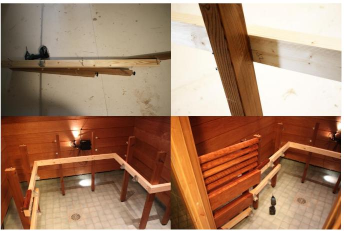
3. Connect the solid frame parts of the lower bench to the lower bench frames. (On the sample frame image, R7, R8 etc.) The screws will be tightened behind the lower bench frame. Do not screw the structure to the wall yet.
