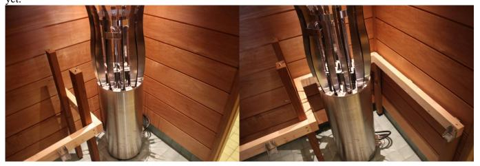
4. Lift the upper bench frames to their places. The upper bench is fitted to the metal pins on the feet by its lower edges. Also assemble the upper frames to each other, do not fasten to the wall yet. Screw the corner curves. The
