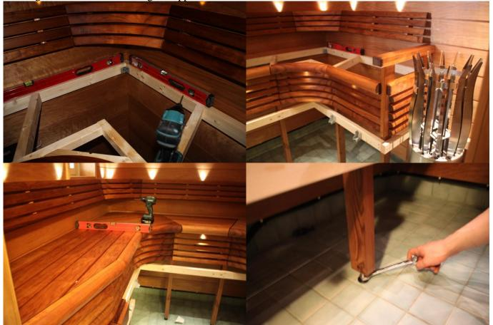
6. Place the spacers of the lower bench in position. If the spacer is on top of the joist hanger, it does not have to be fastened with screws. The joist hanger solution makes sauna cleaning easier, when you can simply lift the frames out of the way during cleaning. PLEASE NOTE! If the solid frames by the walls are long (more than 600 mm), screw them also to the walls, in the same way as the upper benches. Check the straightness with a
