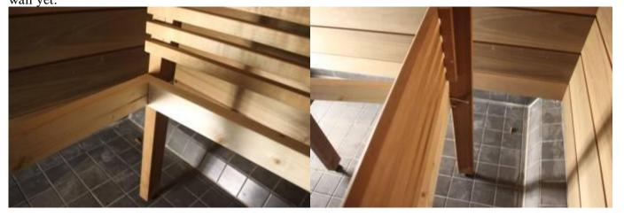
3. Lift the upper bench frames to their places. The upper bench is fitted to the metal pins on the feet by its lower edges. Assemble the upper frames to each other, do not fasten to the wall yet.
