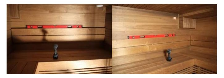
6. Place the spacers of the lower bench in position. If the spacer is on top of the joist hanger, it does not have to be fastened with screws. The joist hanger solution makes sauna cleaning easier, when you can simply lift the frames out of the way during cleaning. PLEASE NOTE! If the solid frames by the walls are long (more than 600 mm), screw them also to the walls, in the same way as the upper benches. Check the straightness with a
