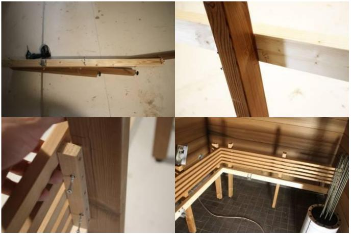
2. Connect the solid frame parts of the lower bench to the lower bench frames. (On the sample frame image, R1, R3, R4 etc.) The screws will be tightened behind the lower bench frame. Do not screw the structure to the wall yet.
